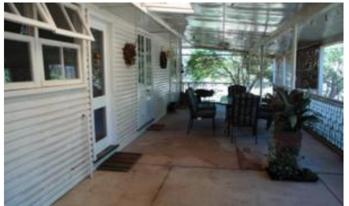
Large enclosed verandah
