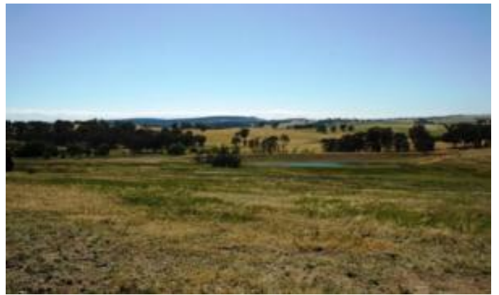
Glen Donald main dam
